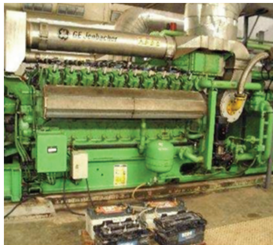
GE Jenbacher Gas Engine - Model J 320
